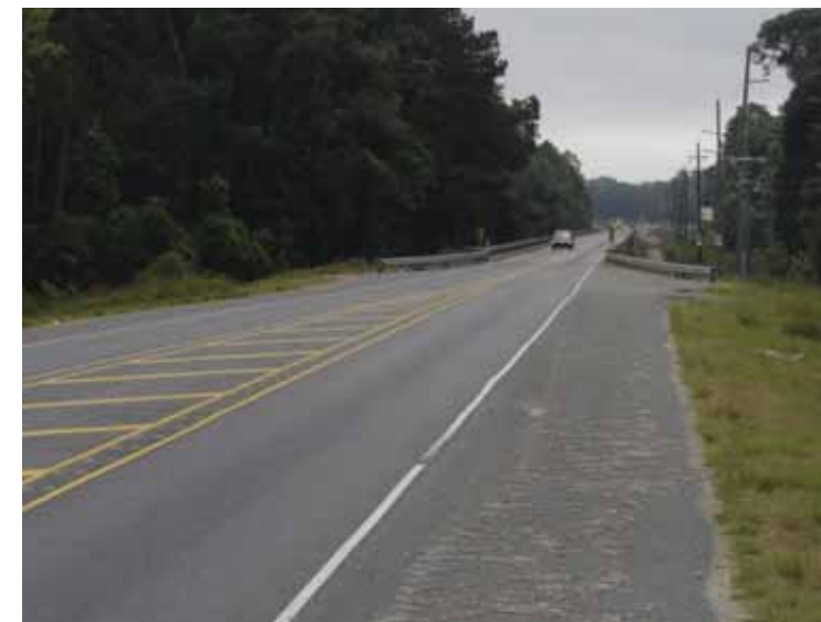
This road shows the wide paved shoulders required in the A2 section. Paved shoulders are a considerable safety improvement and also provide additional facilities for bicyclists.
